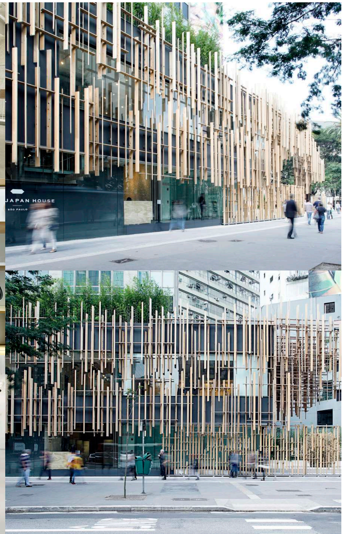
The unique facade of the building is a latticed assemblage ( jigokukumi ) of cypress slats, catching the eyes of passers-by on the avenue. It was assembled by shrine and temple carpenters sent from Japan.
